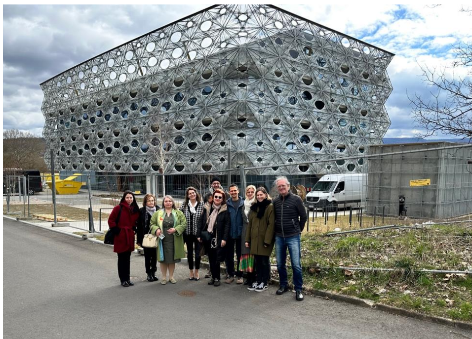
Figure 2: Group photo of the consortium in front of the TEXOVERSUM construction site.
